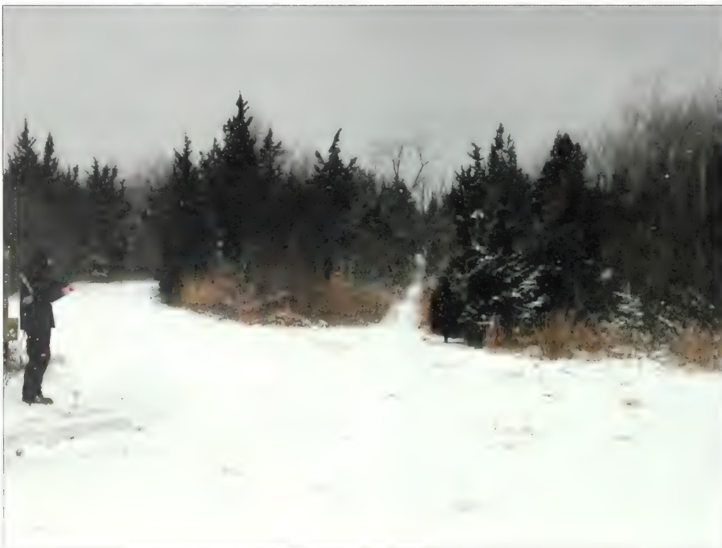
Figure 4.17. View looking northwest at pedestrian walkway, Control Area #1, NIKE radar site. The concrete walkways connecting the control areas and Ready Barracks are presently extant and in fair condition. Some portions of the sidewalks are being covered by encroaching woody vegetation (Olmsted Center, January 2009).
